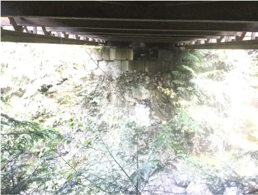
Right Bank Abutment when facing downstream
