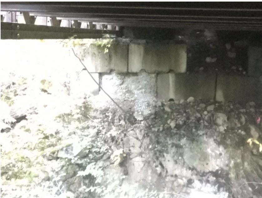
Right Bank Abutment when facing downstream
