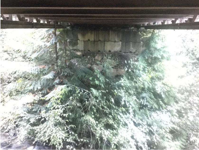
Left Bank Abutment when facing downstream
